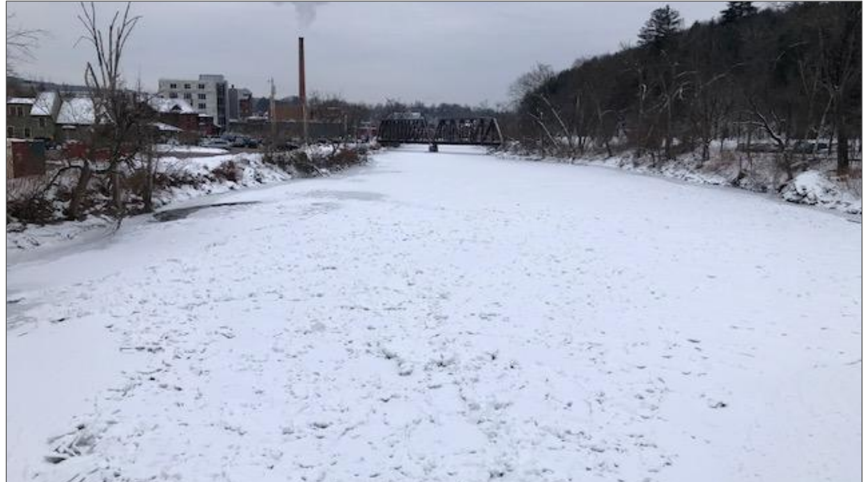
Winooski R. @ Bailey Ave. Bridge, Montpelier, VT (1/13/25)
